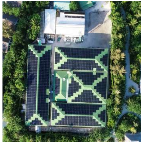
Solar power plant that generates over 478,080 kwh of clean energy for the resort annually.
